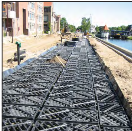
Subsurface Silva Cell & Drain (Use w/ Permeable Surfaces)
