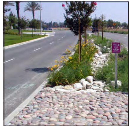
Decomposed Granite/Rock Swale/ Gravel Trench
