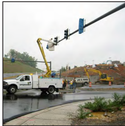
New Traffic Signal at Intersection
