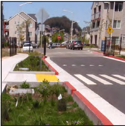
Permeable Curb/Gutter & Curb Openings
