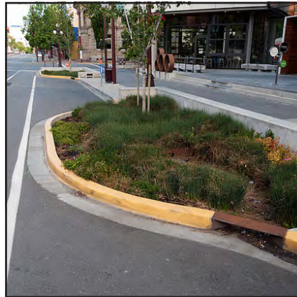
Mid-block Bulbout w/ Bio-retention Soil & Subsurface Drain
