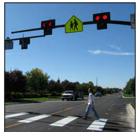
High Intensity Activated Crosswalk Beacon
