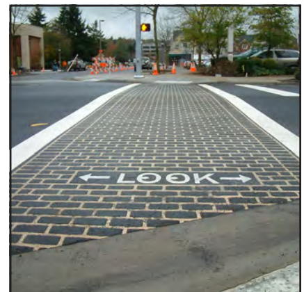
Enhanced Marked Pedestrian Crosswalks
