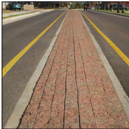
Permeable Paver w/ Subsurface Filtration & Drains
