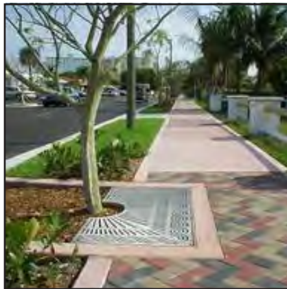
Walkway Over Tree Grate
