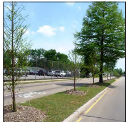
Tree Basin with Bio-retention Soils & Subsurface Drain
