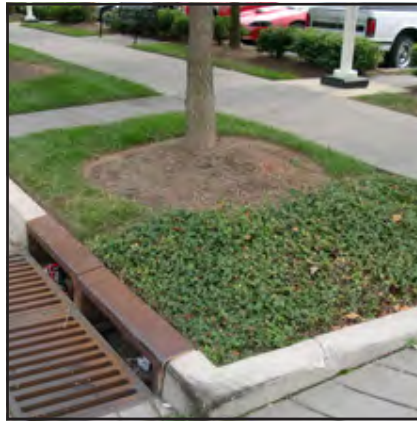
Tree Basin w/ Filters & Subsurface Drain
