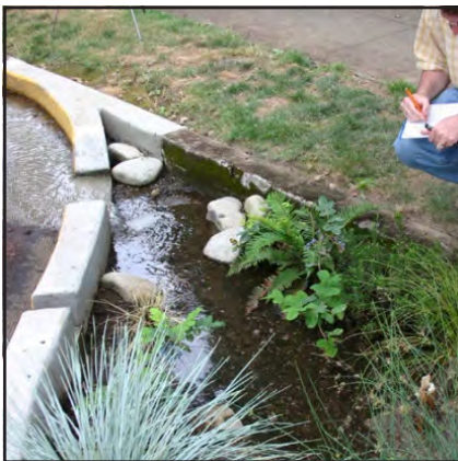
Permeable Curb/Gutter & Curb Openings
