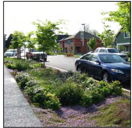
Infiltration Basin w/ Bio-retention Soils & Subsurface Drain
