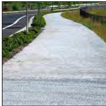
Permeable Asphalt or Concrete
