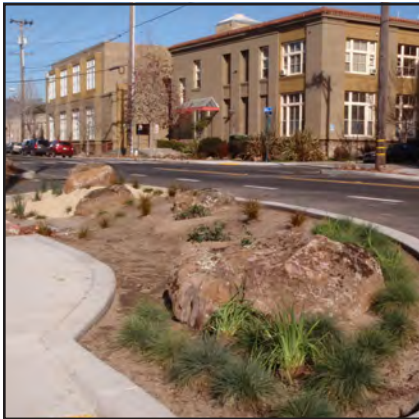
Intersection Bulb-out w/ Bio-retention Soil & Subsurface Drain
