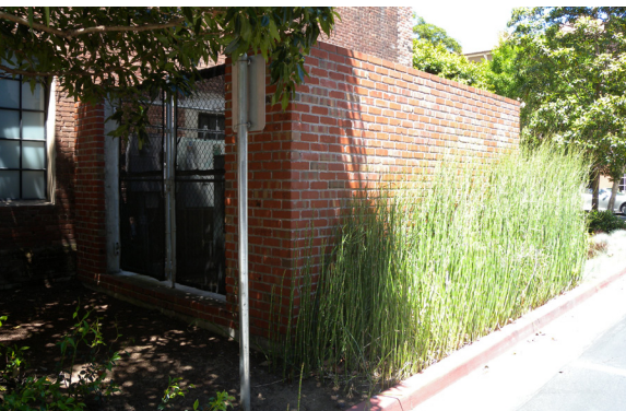
Vines and landscape should be used for screening (top). Screen all visible building equipment, utilities, and trash enclosures in a manner consistent with the building (middle and bottom).
