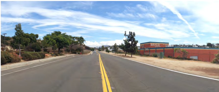
Existing view of Market Street east of Euclid Avenue.
