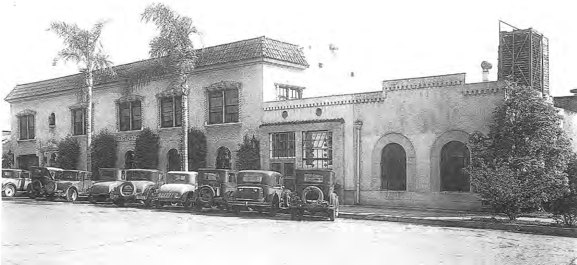
Figure 27. Cramer's Bakery at 1955 Julian Avenue, constructed circa 1924 and pictured here in 1935. (San Diego History Center Photo Archive, #8997)
