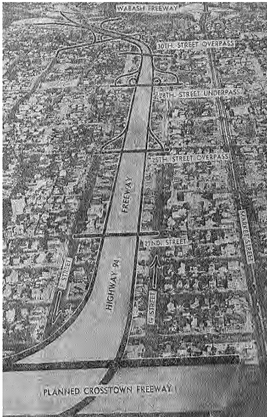
Figure 39. Demolition for Highway 94, through Sherman Heights (San Diego Tribune, 4 January 1957)
