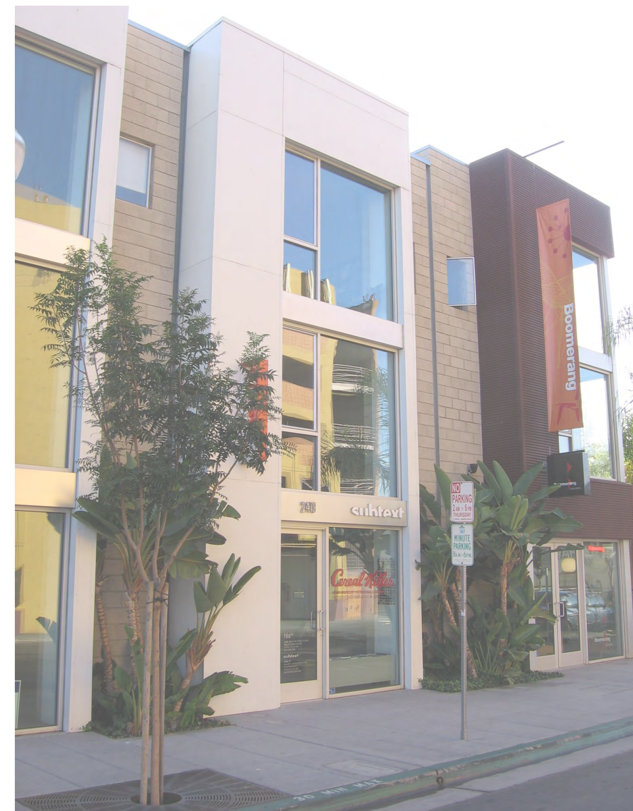
Break down building massing with a change in materials and forms that define a rhythm of bays and sections of a building
