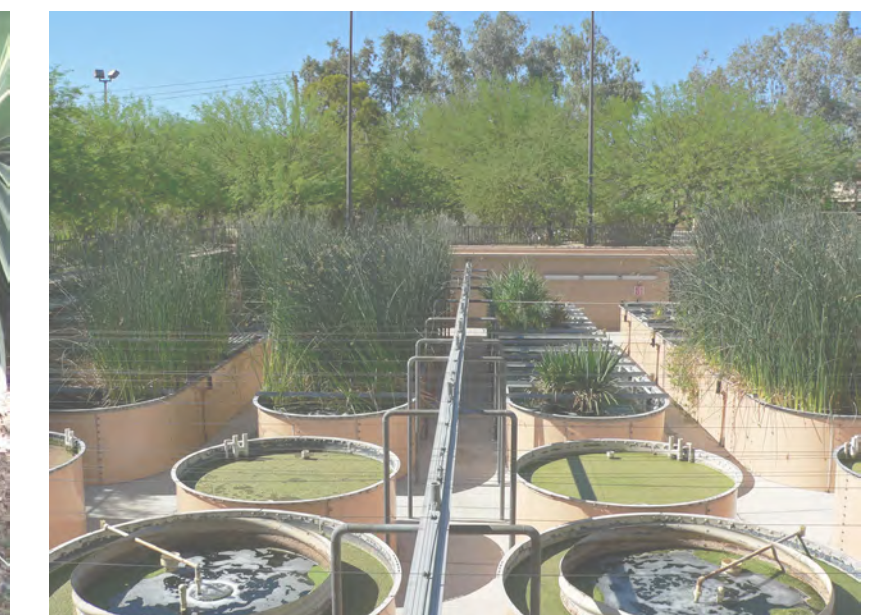
Greywater Tanks or "Living Machines" are one way to recycle and treat wastewater on-site
