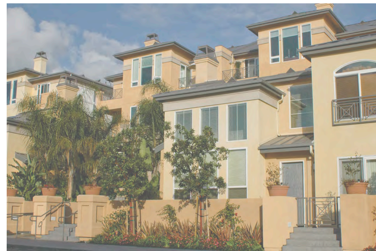
Step back upper stories of a building to diminish the appearance of height on the street
