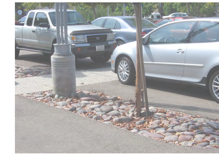
Provide opportunities for natural drainage and permeable paving in all parking areas
