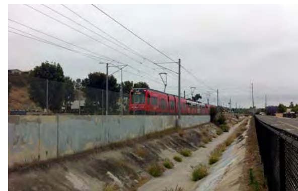
The amphitheater at Market Creek Village (top) and the path east of Euclid Avenue (middle) show the promise of creekside enhancements. Many creek segments present challenges (Imperial Avenue, bottom).
