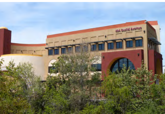
Prominent buildings include the Elementary Institute of Science, St. Rita's, and Jacobs Center.
