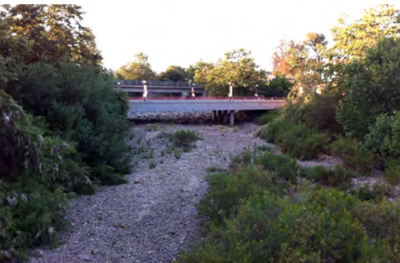
Stormwater swales and preserved open space (top and middle) allow water to infiltrate, preventing polluted runoff from entering streams.
