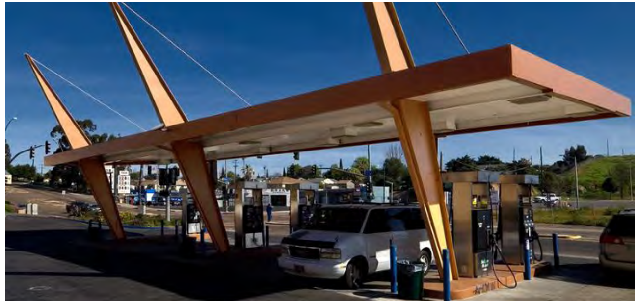
Johnson's Wilshire Gas Station on Market Street, built in 1962, retains distinctive characteristics of Googie architecture and is listed on the City's Register of Historical Resources.
