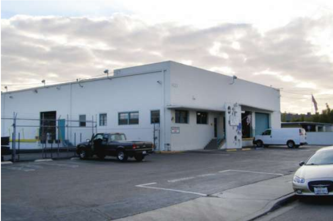
Figure 7. Typical industrial building in project area, 4530 Mission Gorge Place.
