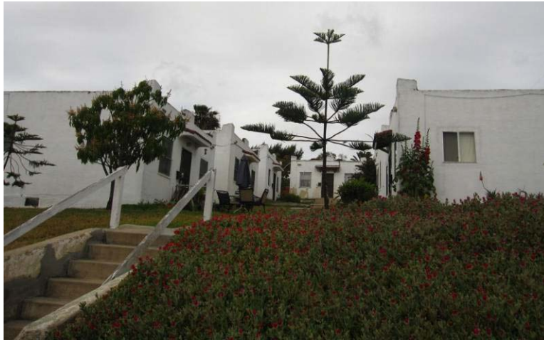
407 W. San Ysidro Blvd, 1928 (Source: Page & Turnbull, April 2010)
