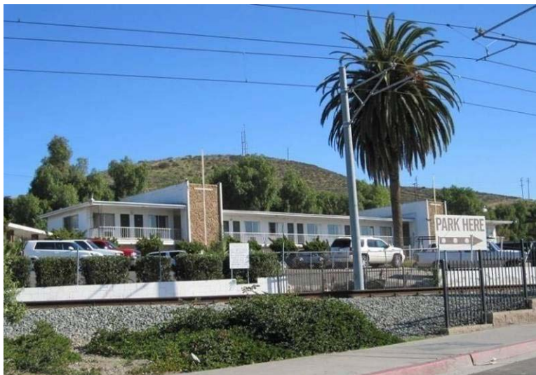
701 E. San Ysidro Boulevard, Motel near Port of Entry, ca. 1960s. (Source: Page & Turnbull, April 2010)
