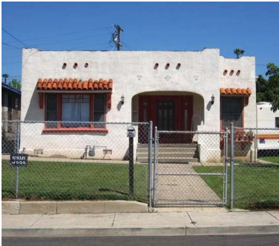
159 Hall Avenue, 1923. (Source: Page & Turnbull, Jan 2010)
