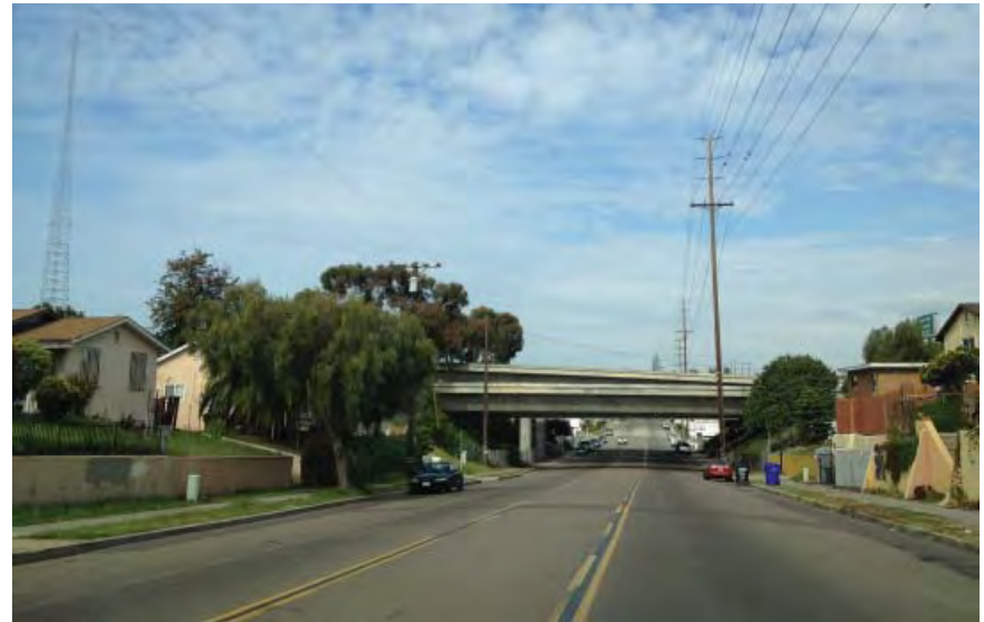
View west on National Avenue, with SR-15 overpass in sight
