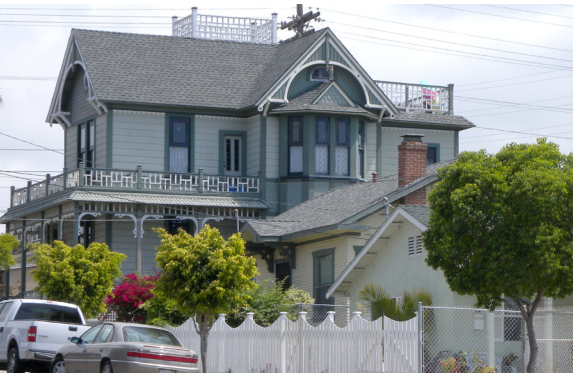
Villa Montezuma and Hollington House (top and bottom) are listed in the National Register of Historic Places and the San Diego Register of Historical Resources, respectively.
