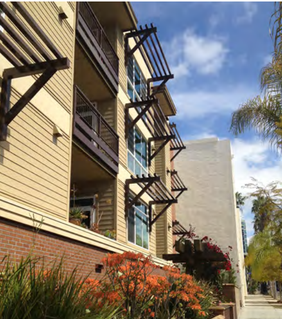
Landmarks (such as the Villa Montezuma) are cherished symbols of community pride and character (top). Windows positioned to maintain sight lines toward street, and clearly visible entryways help create security through design (bottom).
