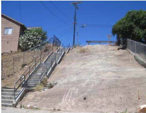
Branches of Chollas Creek create terraces in the land mass and steep drop-offs, as shown east Bancroft Street.
