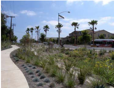
Permeable pavers and landscape areas installed on Logan Avenue near 43rd Street allow for stormwater infiltration which reduces flooding potential and runoff.
