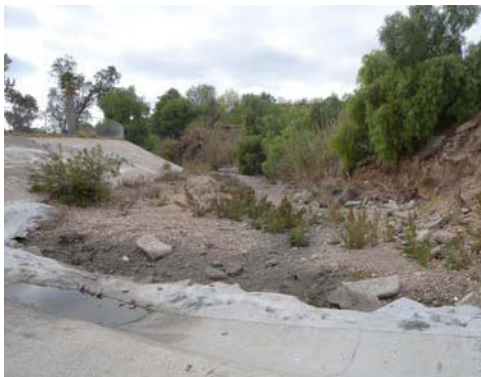
Improvements to Chollas Creek were made as part of the Imperial Marketplace development (top). Planned improvements to the creek segment between Greenwood Cemetery and the YMCA (middle and bottom) are detailed in the South Branch Implementation Program.
