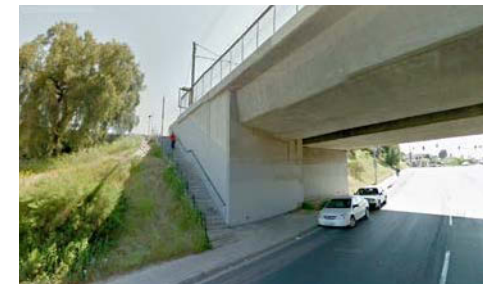
25th Street Trolley Station (top). Stairs at 32nd Street Trolley Station (bottom).
