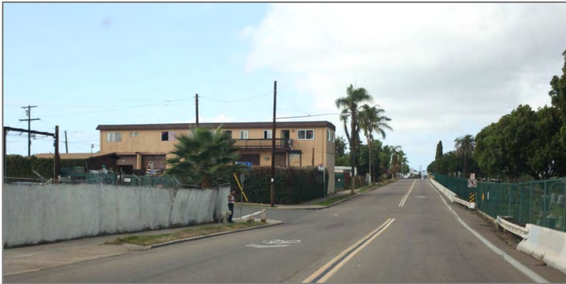
Class III Bike Route (with Sharrows) along Imperial Avenue, between 36th Street and 40th Street.
