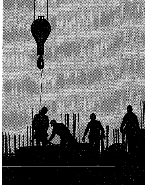
Capital improvements under construction
