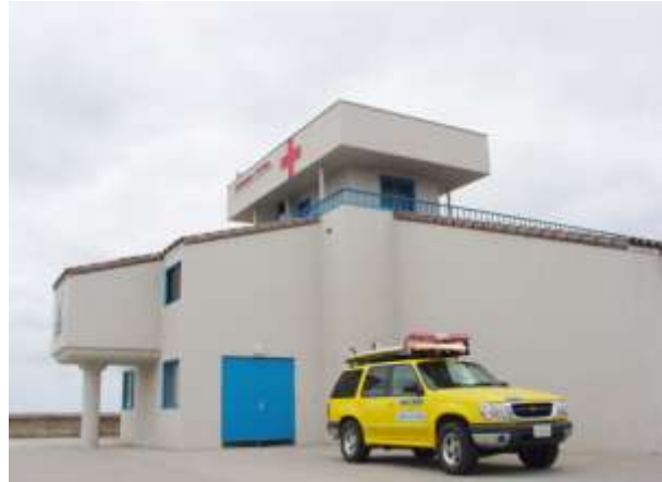
Fire-Rescue Mission Beach Lifeguard Station
