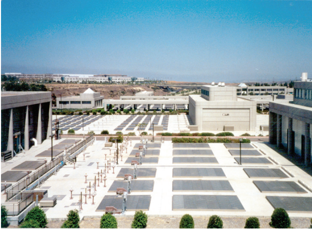
North City Water Reclamation Plant Opened 1997 Design capacity: 30 MGD 24 MGD available for distribution after plant processing use
