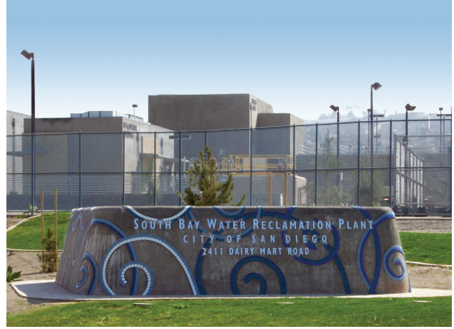
South Bay Water Reclamation Plant Opened 2002 Design capacity: 15 MGD 13.5 MGD available for distribution after plant processing use
