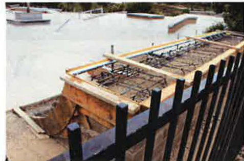
One of several ramps under construction at Black Mountain Ranch Skate Park.
