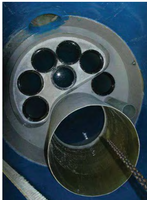
The depth of sediment and oil can be measured from the surface by using a sediment probe or dipstick tube equipped with a ball check valve and inserted through the 30-inch maintenance access pipe. This large port provides convenient access for inspection and vacuum removal of water and pollutants.
