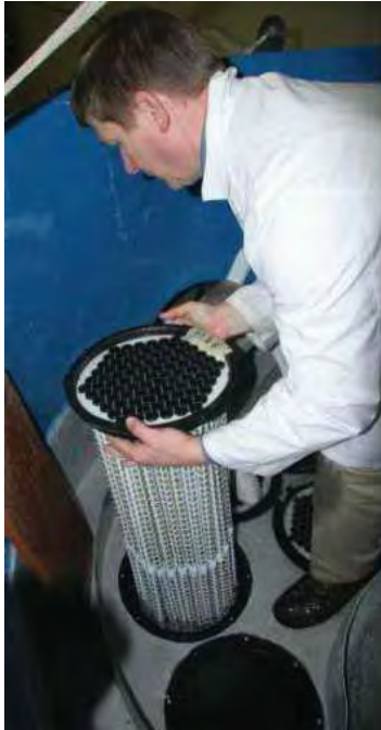
Lightweight Jellyfish filter cartridges are easily inserted into and removed from the cartridge deck by hand. The top view schematic (above right) and top view photo (below right) depict the 6-ft diameter system. Note the 6 standard cartridges enclosed by the kidney-shaped backwash pool weir. A single draindown cartridge is located outside the weir.
