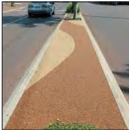
Permeable Concrete w/ Sand Filtration & Subsurface Drain
