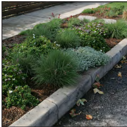
Rain Garden with Bio-retention Soils & Subsurface Drain
