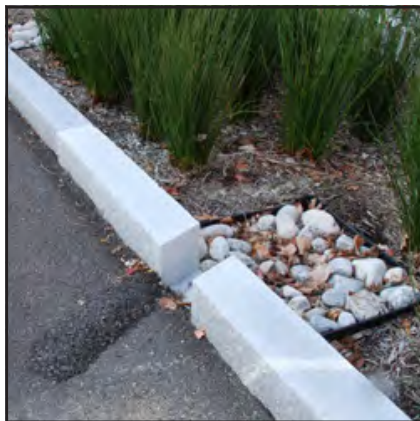
Permeable Curb/Gutter & Curb Opening
