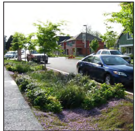
Infiltration Basin w/ Bio-retention Soils & Subsurface Drain
