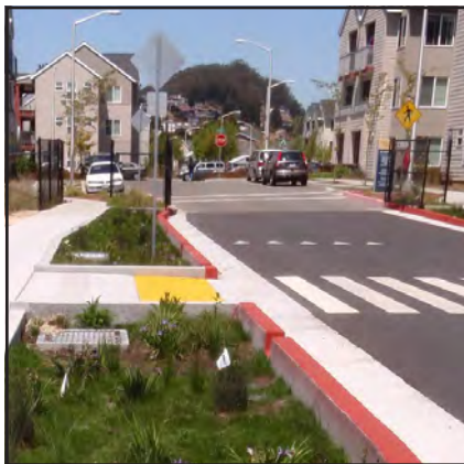
Permeable Curb/Gutter & Curb Openings
