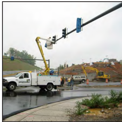
New Traffic Signal at Intersection
