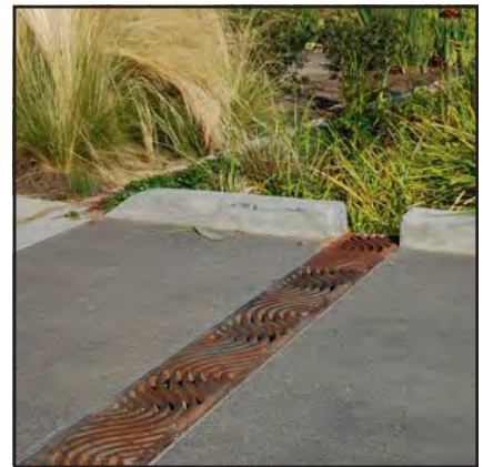
French Drain with Grates
