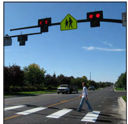
High Intensity Activated Crosswalk Beacon
