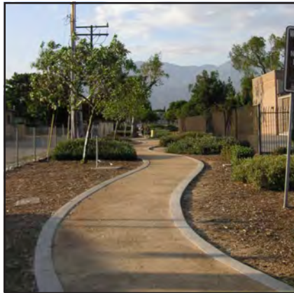
Compacted Decomposed Granite Walkway
