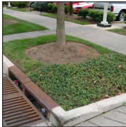
Tree Basin w/ Filters & Subsurface Drain
