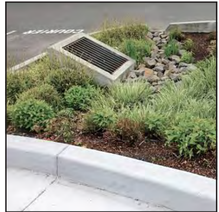
Bulbout as an Infiltration Basin w/ Bio-retention Soils & Subsurface Drain
