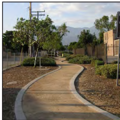
Compacted Decomposed Granite Walkway
