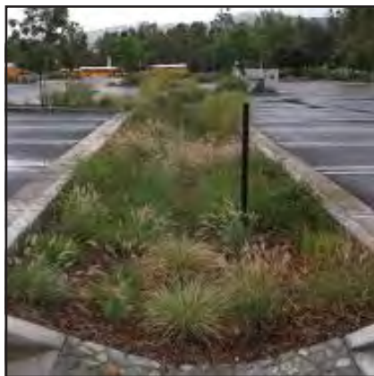
Infiltration Basin w/ Bio-retention Soils & Subsurface Drain
