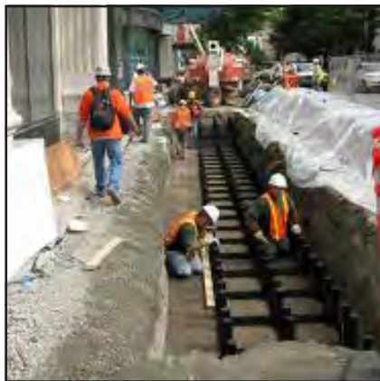
Subsurface Silva Cell Drain (Use with RS2.1)
