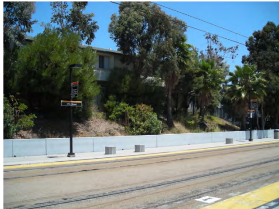
Transit Station at 47 th Street
