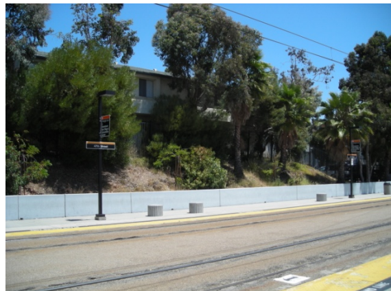
Transit Station at 47 th Street
