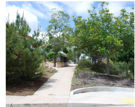
Streets with wide parkways are candidates for stormwater infiltration using landscaped swales.
