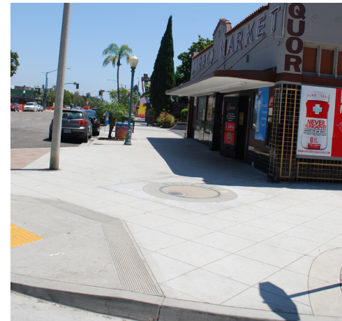
Streetscape renovations that include pedestrian improvements such as the 25th Street Renaissance Project can rehabilitate aging infrastructure and improve the pedestrian experience.
