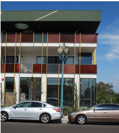
Historic "acorn" style street lighting not only improves safety for pedestrians, vehicles and properties at night but also provides a unifying character statement within the community.
