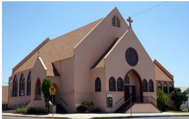
The Christ United Presbyterian Church, located on 3025 Fir Street, has been identified as a potentially significant individual resource.
