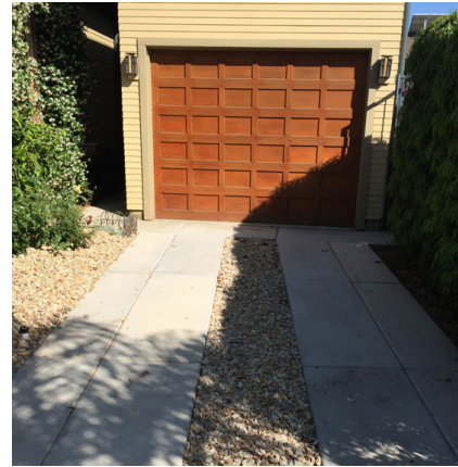
Residences upstream from natural drainages can contribute to water quality improvement by reducing the amount of impervious driveway area.
