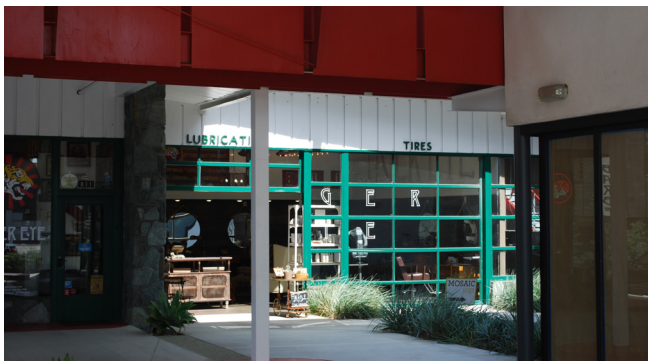
This development responds to its site context through the reuse of an old service station building.
