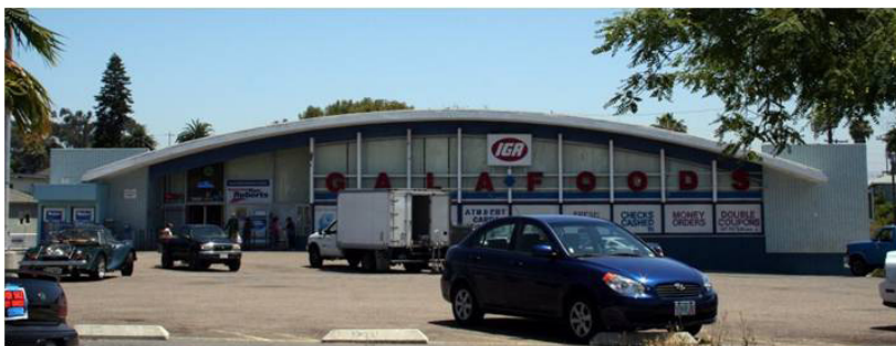
The property on 2001 Fern Street, built in 1960, has been identified as a potentially significant individual resource related to the Era of Transitions Theme (1930-1990).
