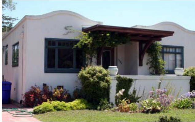
The property on 1345 Granada Ave. is designated as HRB site #612 and was designed by Master Architect Irving Gill in 1909.
