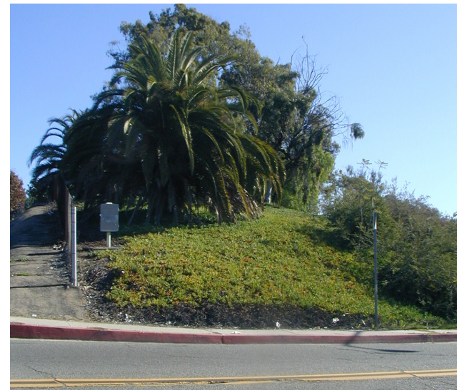
Physical separation from auto travel lanes reduces freeway noise on adjacent land uses. A landscaped berm is used here at an interchange with State Route 94.
