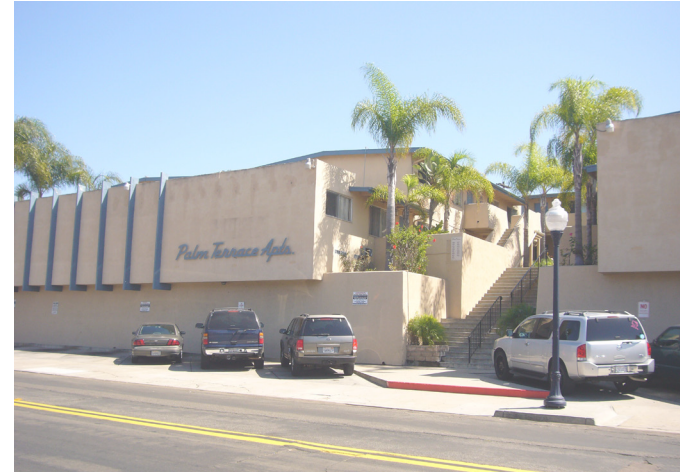
BEFORE: Existing Apartment Building
