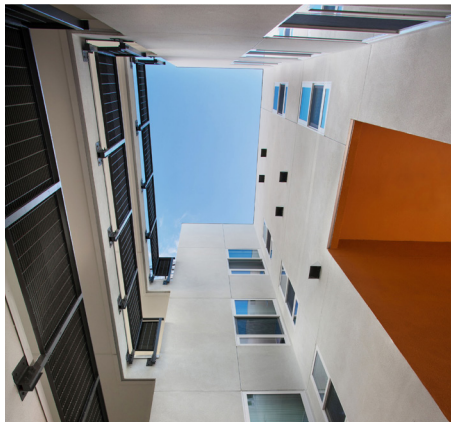
Light wells and light courts are an excellent way to bring natural light and ventilation into a building and make the interior environment more livable.
