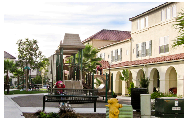
Building windows and entrances should face playgrounds, common areas and shared open spaces to activate them and provide plenty of “eyes on the open space”
