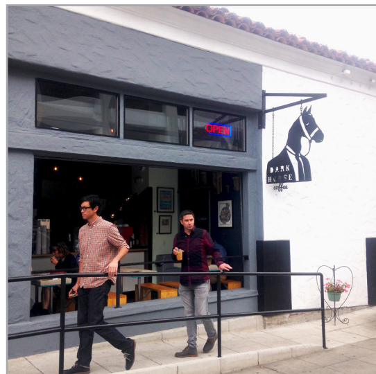
Older buildings can be retrofitted to create new indoor - outdoor experiences.
