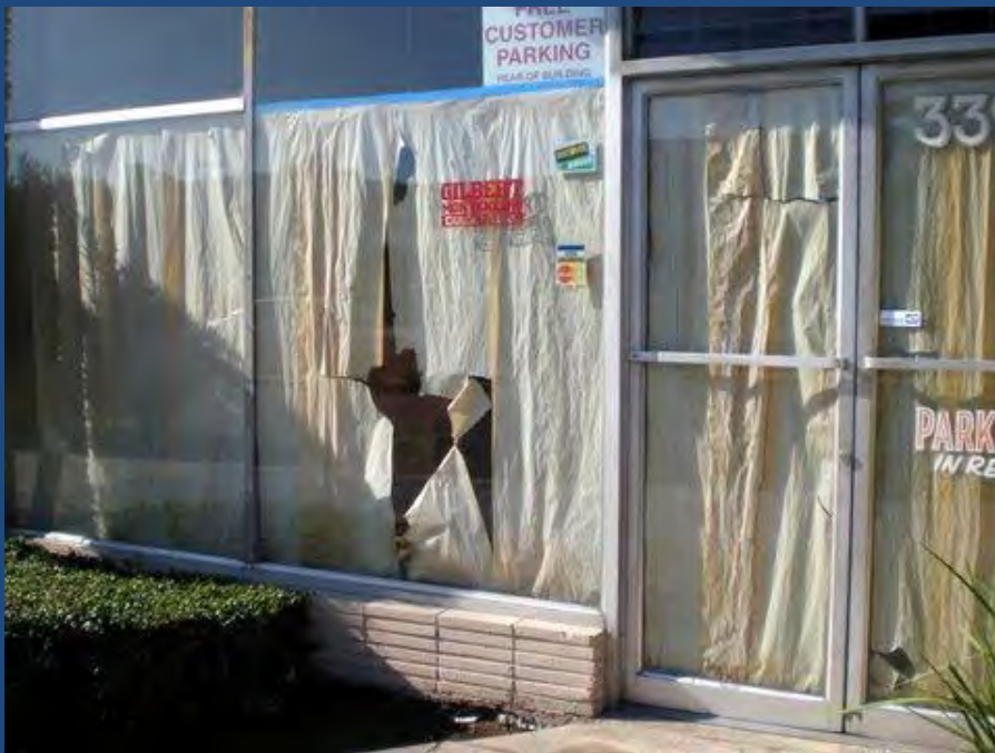
3300 block 30 th Street. Ugly window covering for empty space.
