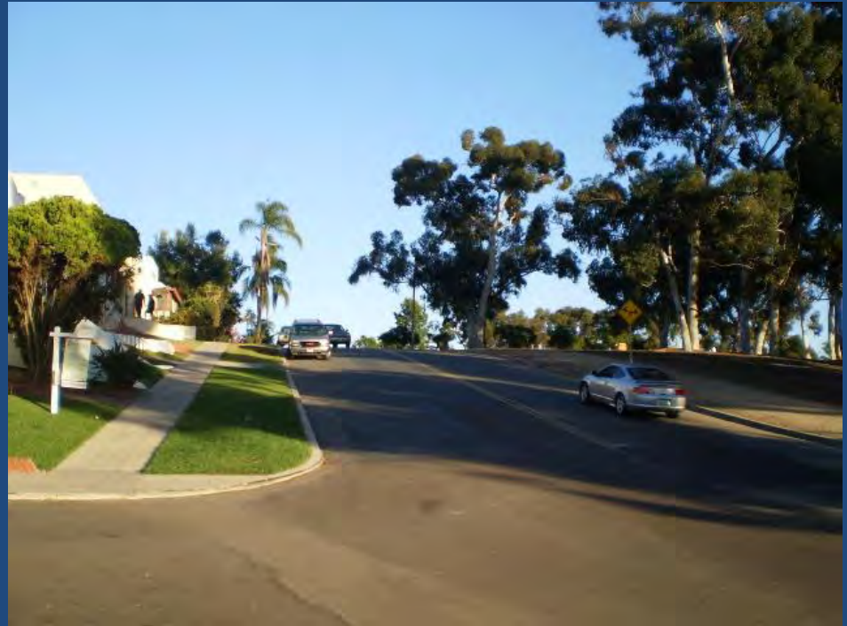
Dangerous vertical curves with no traffic calming for pedestrians.
