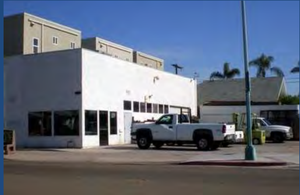
3700 block 30 th Street Box architecture; no buffer for car/equipment parking.
