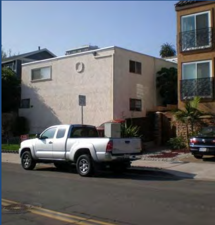
Florida Street. MF Box architecture. Tiny windows.
