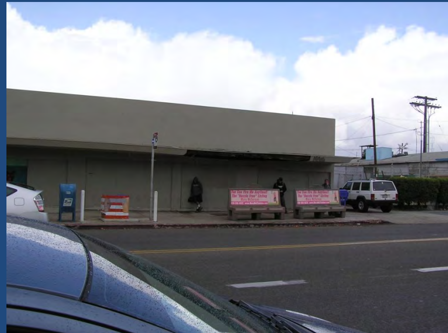
Pat's at Upas/30th - façade is deteriorating and unsafe at bus stop.
