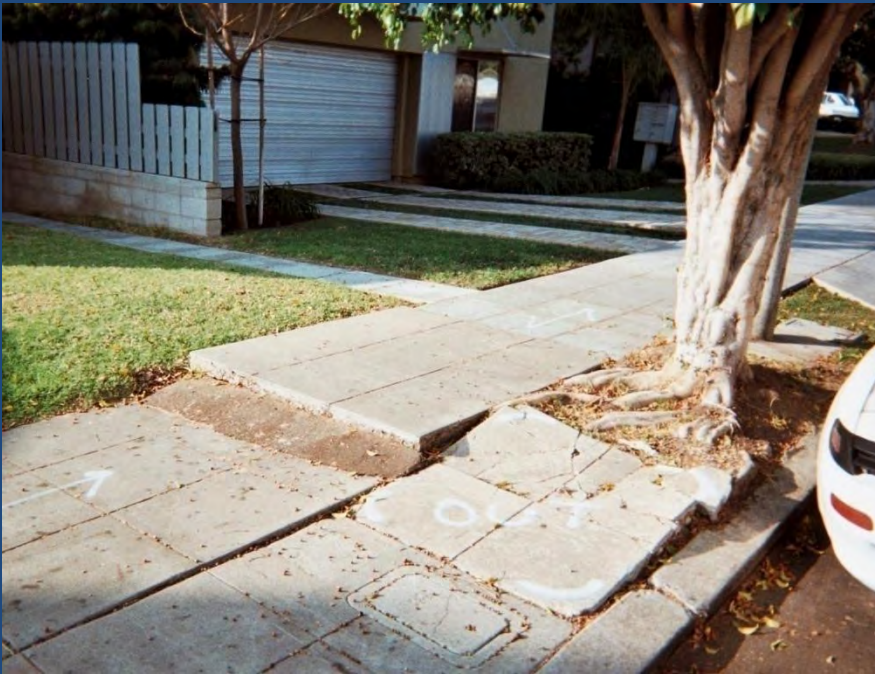
4024 Hamilton - dislike dangerous sidewalk transition
