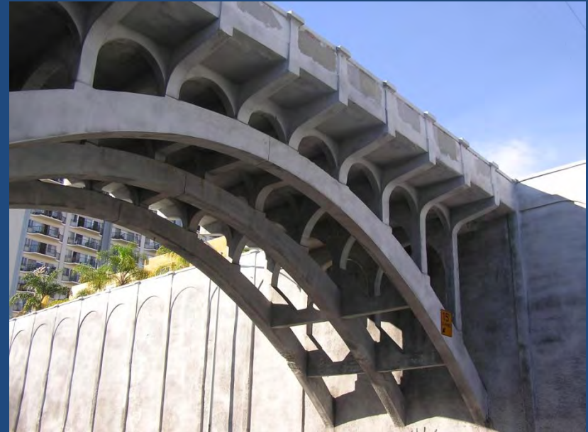
Georgia Street Bridge (University Avenue)
