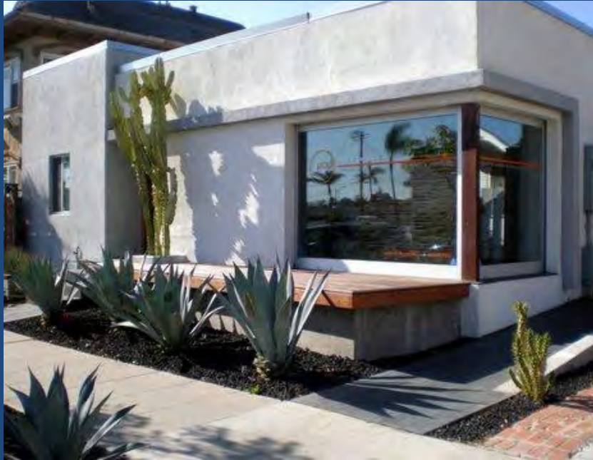
3700 block 30th street. Compatible contemporary remodel.
