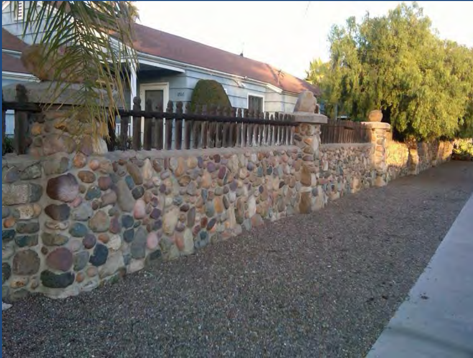
Rockwork pillars & wall from Mission Cliffs Gardens
