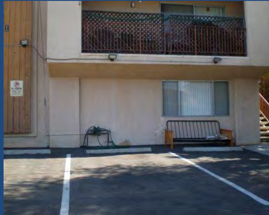
3361 Dale Street. MF with exposed wiring and dilapidated furniture.
