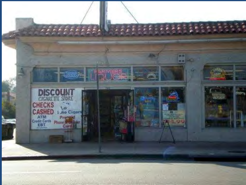
2045 University Avenue. Sign code violation.
