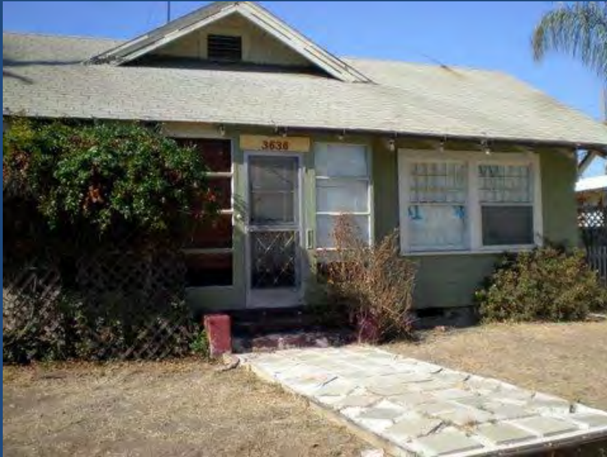
3636 30 th Street. Unkempt house/papered windows on commercial corridor.
