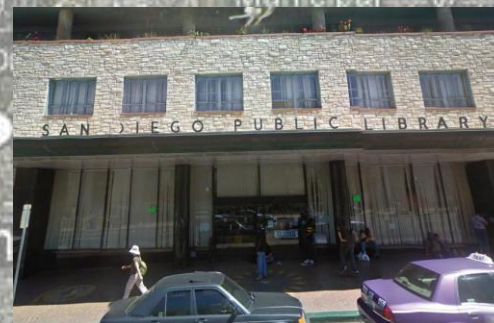
Main Central Library – 144,000 SF
