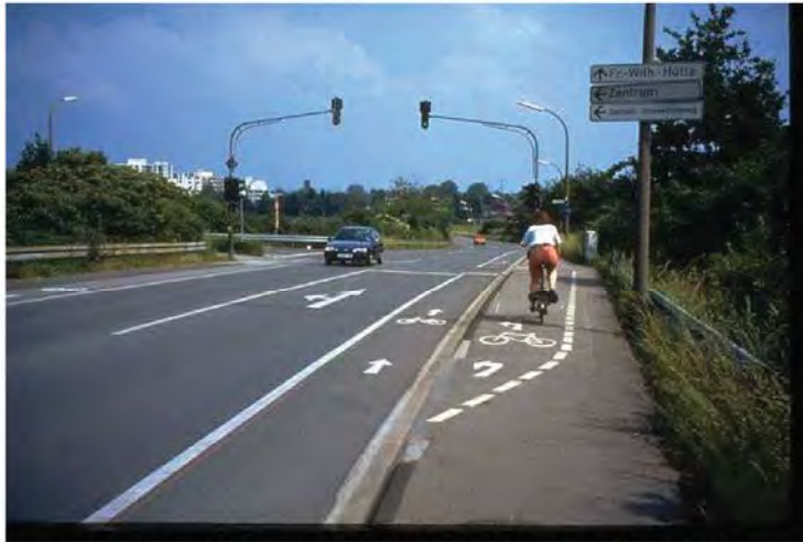
Troisdorf, Germany: Bicyclist directed to right to make a "box left" turn.
