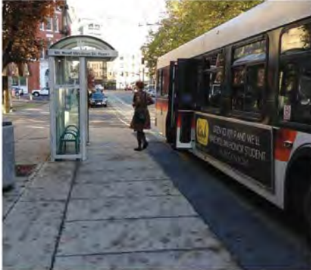
Having multiple vehicle types sharing a platform impacts both platform height and length. This image shows a bus sharing a 10 in. near-level streetcar platform in Portland.
