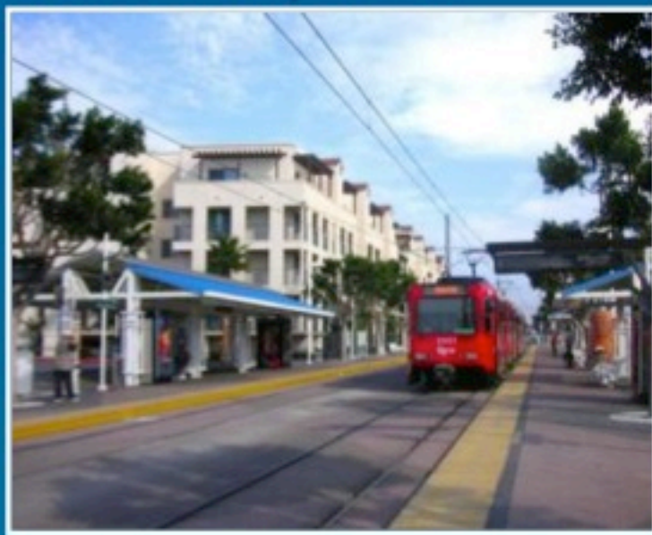
Morena/Linda Vista Trolley Station
