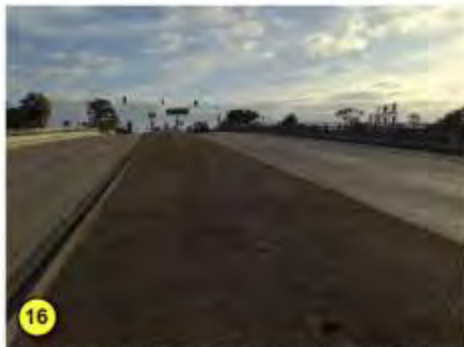
16 The median on Tecolote over the tracks / freeway is very wide and could be reduced to make room for bike lanes
