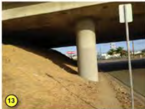
13 No walkways exist under Tecolote at West Morena Blvd.
