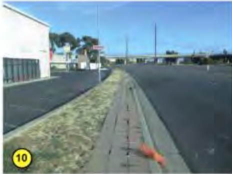
10 Some areas contain walkable surfaces but they are too narrow and do not meet ADA requirements
