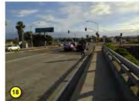
18 This segment of Tecolote does not require two through lanes and two left turn lanes
