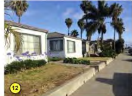
12 Though not high density, some of the courtyard housing is unique and are moderately dense
