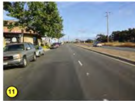
11 Some excessive lane widths and median widths exist that could be reclaimed to make room for bike lanes
