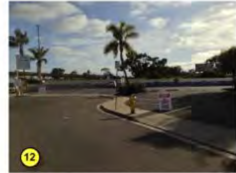
12 Knoxville could be made to connect with West Morena Blvd. if grading and right of way is acquired
