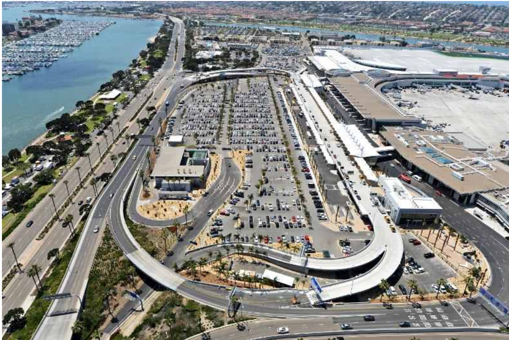
QC Southwest worked on multiple projects on the airfield, in the terminal and on the dual-level roadway.
