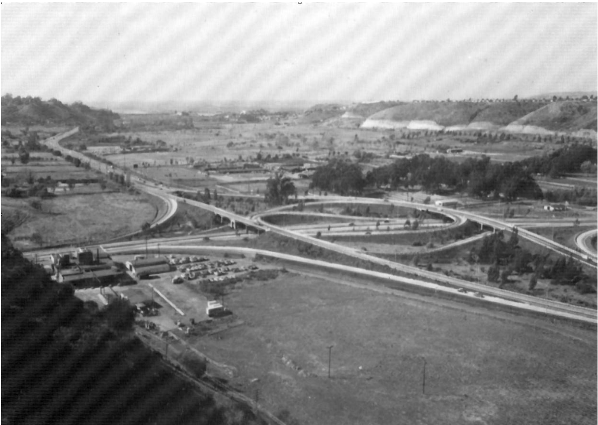
Cloverleaf with dairy on left side looking west from Madison Street, November 1954
