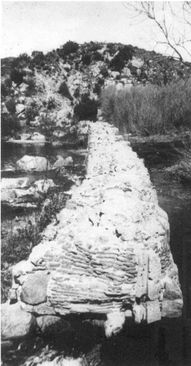
Remaining structure of the old mission dam built in the 1700s to provide water for irrigation
