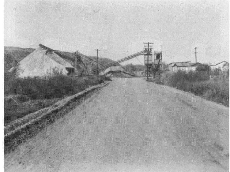
American Sand Company, just north of Twain and Powers Streets, December 1954
