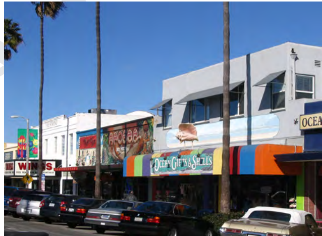
Newport Avenue Commercial District
