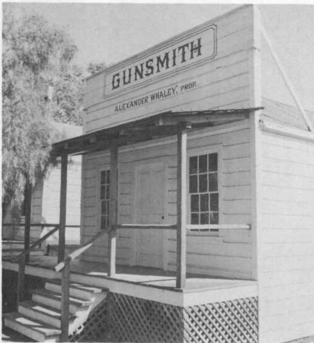
One of the characteristic small buildings with covered entrance (center) and false front which usually indicated a business establishment. Note double-hung wood sash, wood siding, pitched roof (usually shingled).
