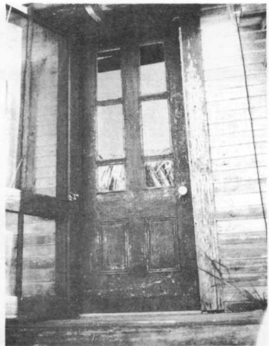
Note wood siding, door and windows and trim, and small cornice effect carried on brackets.
