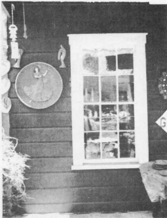
Note wood siding, door and windows and trim, and small cornice effect carried on brackets.
