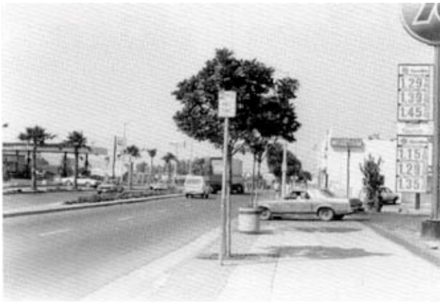
Portion of San Ysidro Boulevard widened in 1989
