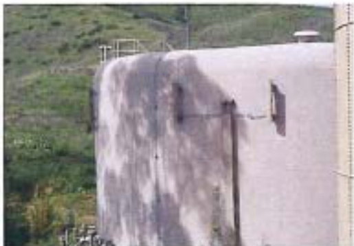
SITE PRIOR TO INSTALLATION
