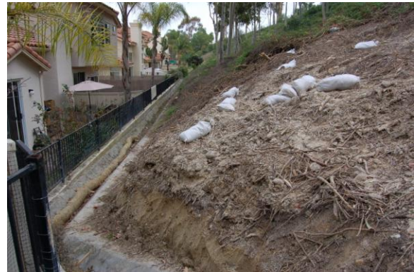
View east of toe of shallow slope failure.
