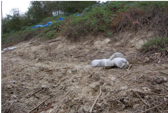
View east of headscarp of shallow slope failure.
