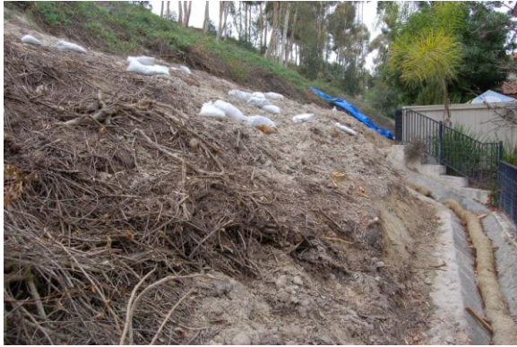
View west of toe of shallow slope failure.
