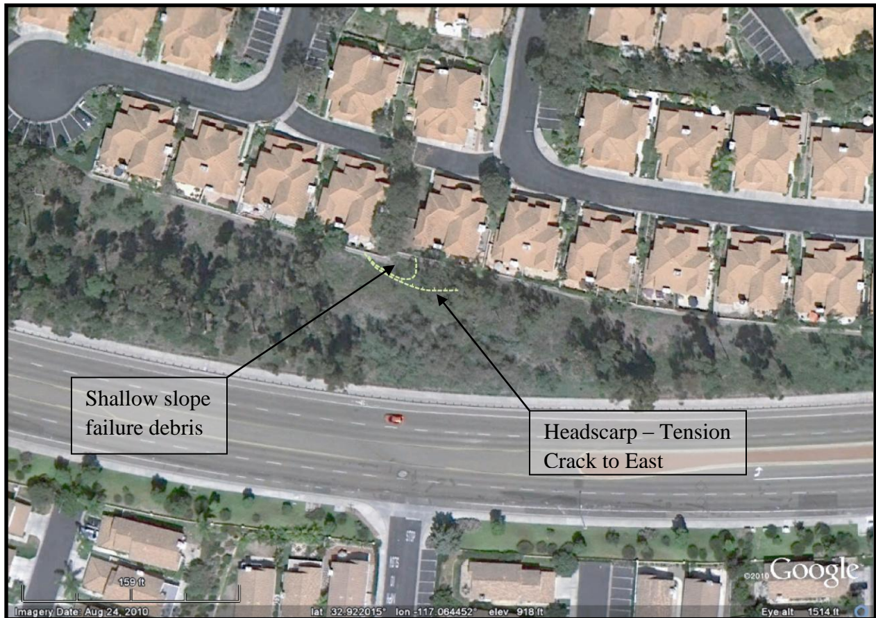
Figure 2. Aerial photograph showing approximate area of shallow slope failure.
