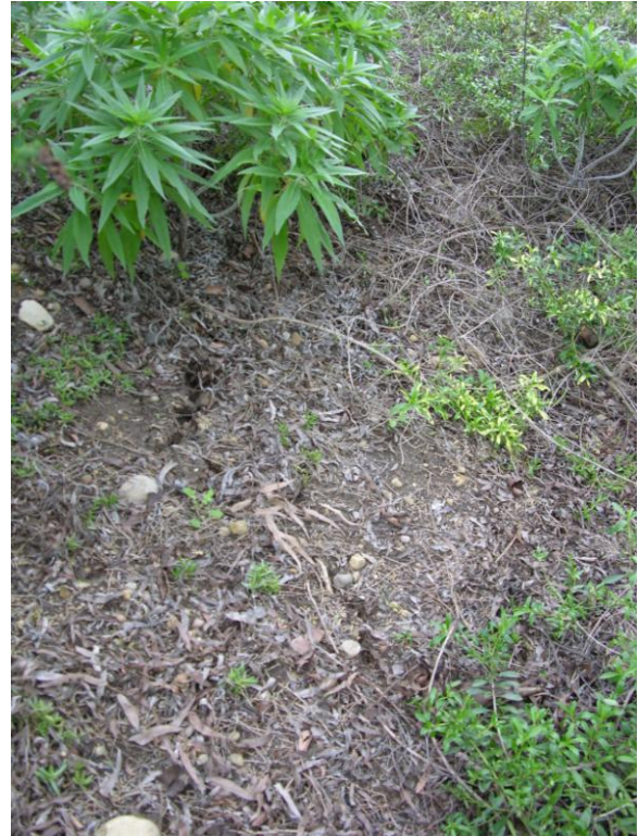
Tension crack at east end of slope failure.
