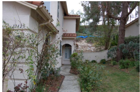
View south between 12425 Caminito Briosso and 12389 Caminito Vibrante of shallow slope failure.
