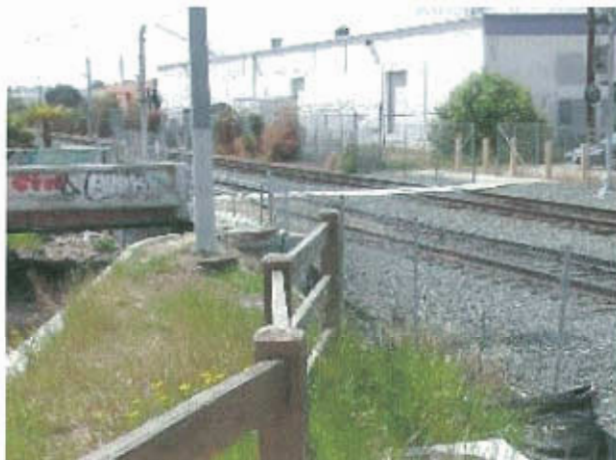
Area of possible connection between 54 th Street and Potter's Tract trail
