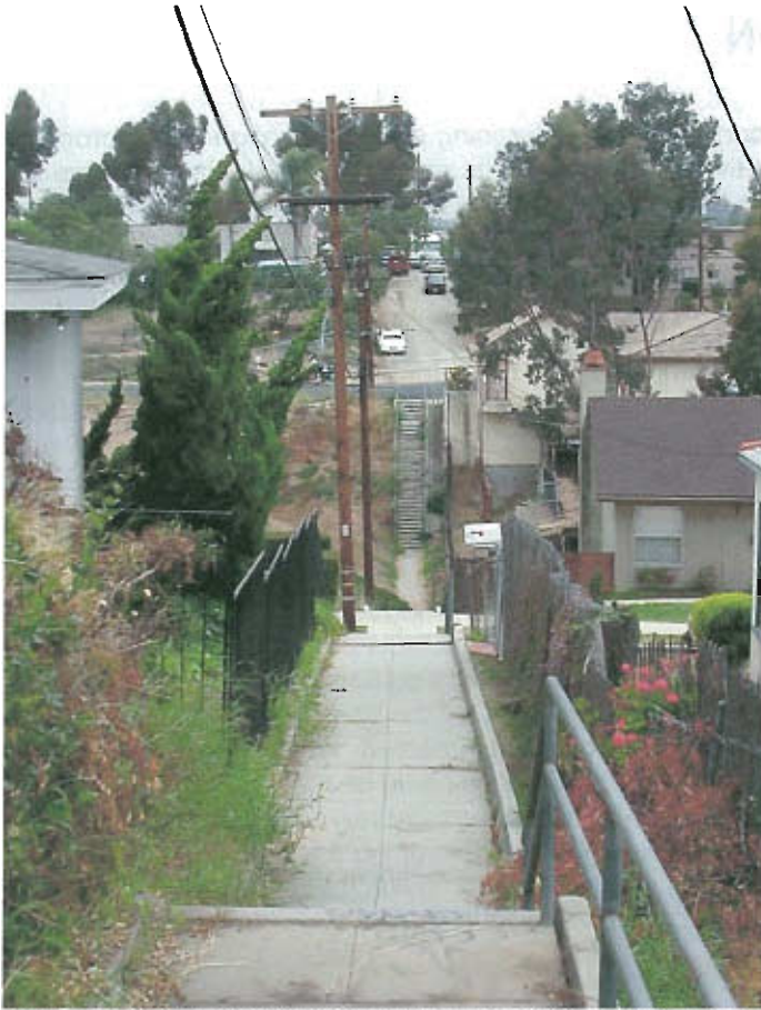
Sewer right-of-way/pedestrian path leading to Churchward and Vista Grande apartments on top of the hill
