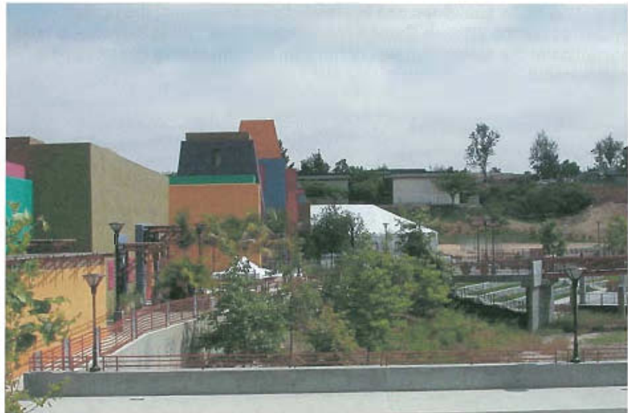
Chollas Creek at Market Creek Plaza
