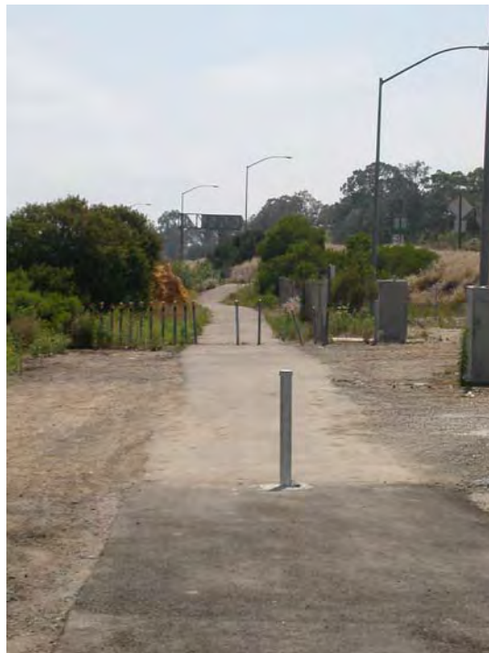
Beginning of Bicycle Path at Federal
