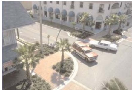
Pop-outs and decorative paving at intersection
