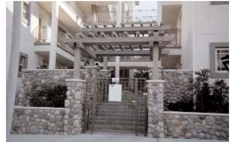
Clearly defined entrance and separation of private and public space
