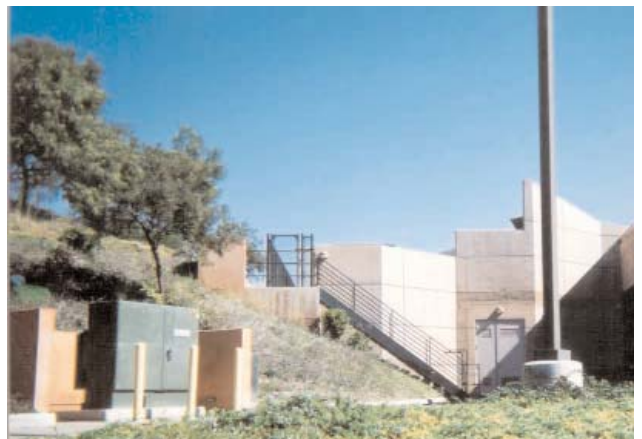
Building built into existing hillside
