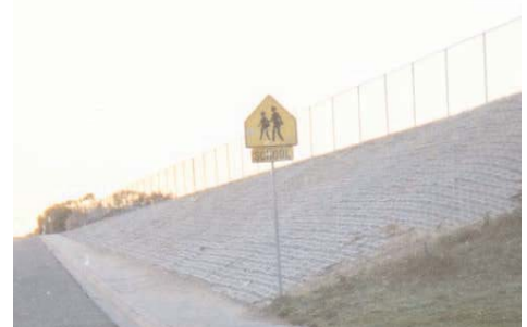
Paved slopes - not desirable
