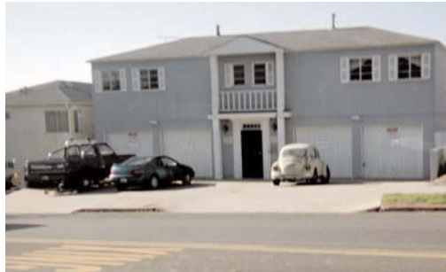
Too many curb cuts disrupt pedestrian flow
