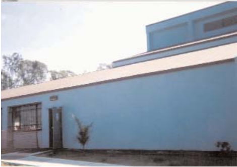
Long, blank walls should be avoided
