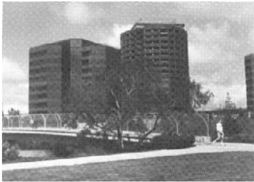
Good example of landing area at the end of a pedestrian overpass.
