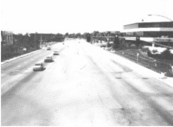
The wider the street the greater the need for landscaped medians to break the vast expanses of asphalt.
