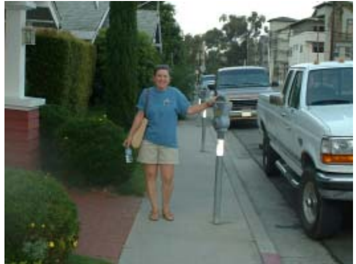
Narrow sidewalks are squeezed further by parking meters, which could be consolidated.
