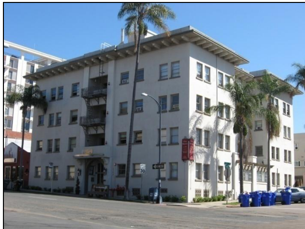
Figure 14. Kirkland Apartments, 2309 5 th Avenue, HRB #483 Source: CPCI Staff
