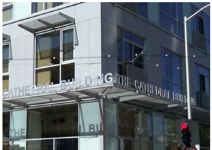
Residential signage should be simple and discreet and not overpower building design.
