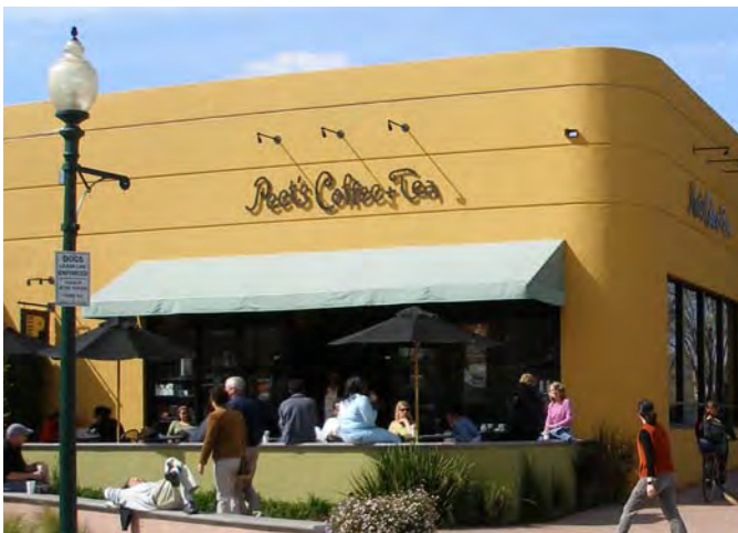
Signs should be integrated with overall building design with a simple and clear message.
