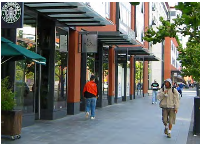
Ground-floor uses should be active, on level with the sidewalk, and punctuated with design elements that are in scale with the pedestrian realm.
